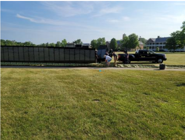
Wall being constructed at Lawton Loop, Lawrence Indiana.
